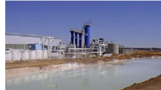
Side view of Takata Corp's 23,000tpa salt removal capacity plant in South Australia for production of high purity magnesium metal feedstock and byproducts from seawater brines using Salpro .
